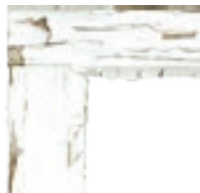
✗ Old painted wood exterior.
